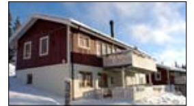
MÅRDEN Apartments varying in size and number of beds. More details at skistar.com
